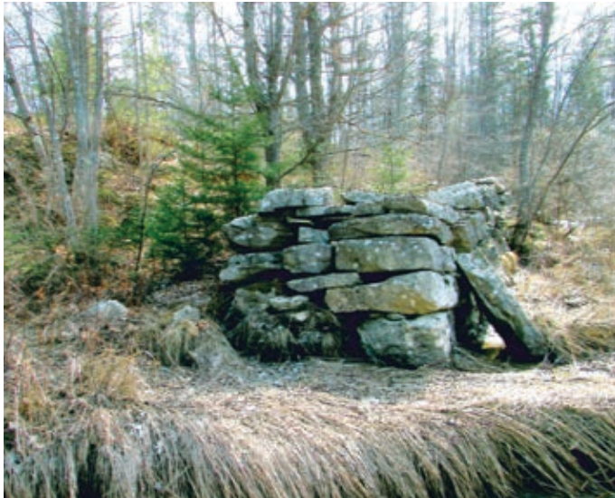
Northeast end of foundation next to Grist Mill, Fulling Mill and the Dye House.
