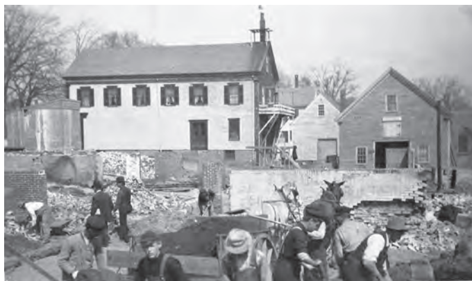
Aftermath of the fire of 1909 that burned the Clark and Mallet Blocks on Main Street between Bow and Mechanic Streets.
