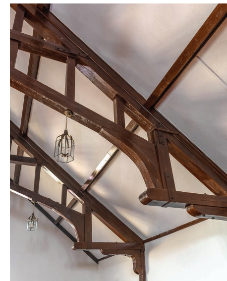
Hand-hewn trusses supported by knee braces.
